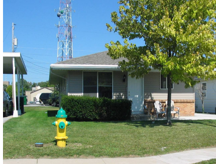
Shown above is one of the six rental rehabilitation projects completed in FY 2006.
